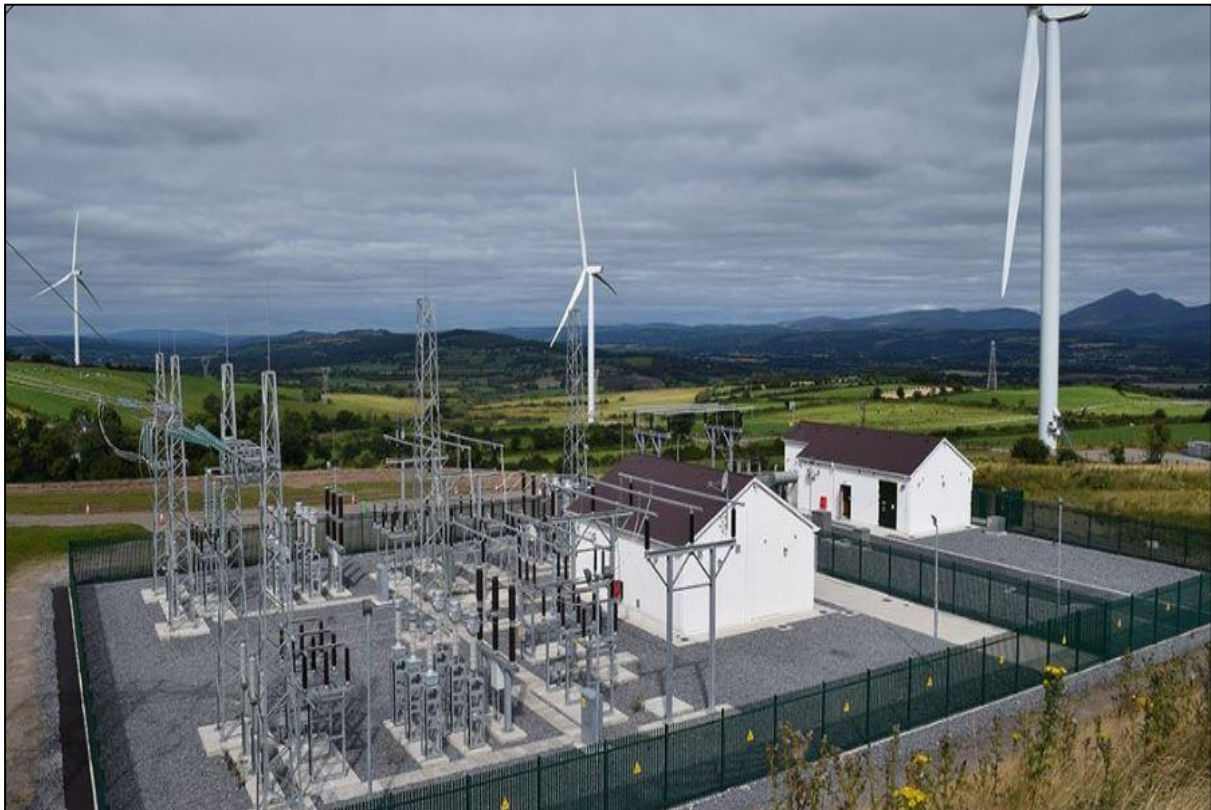
Figure 5: Typical 110kV AIS Substation
